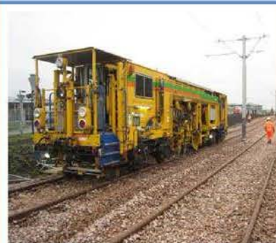
Tamper on Section 7
