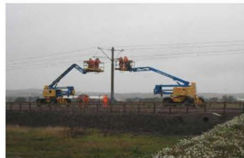
Overhead Line Installation
