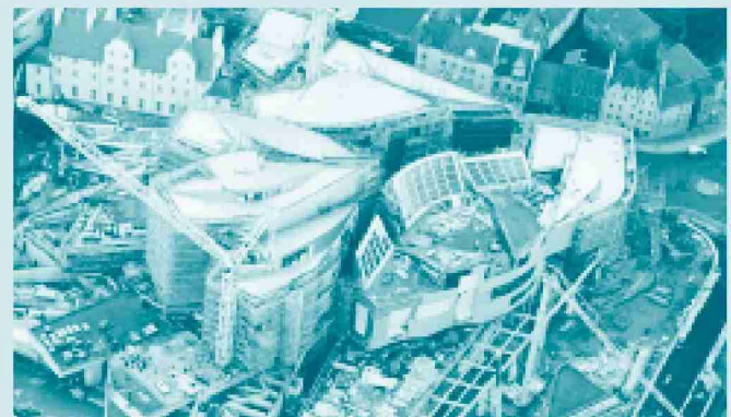
Main building complex (looking from south)
