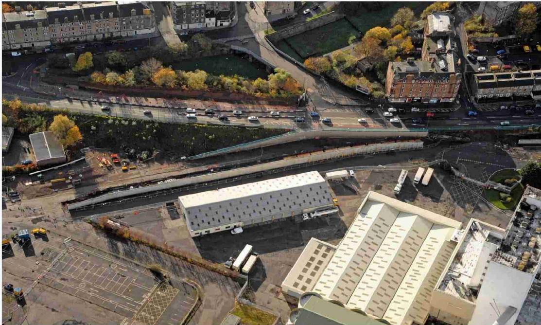
Picture 01 Section 1A Lindsay Road Retaining Wall
