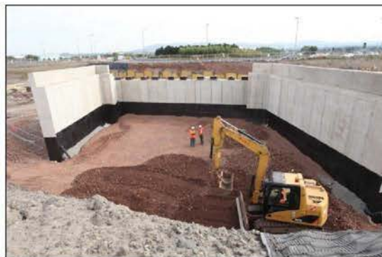
Gogar Depot Access Bridge
