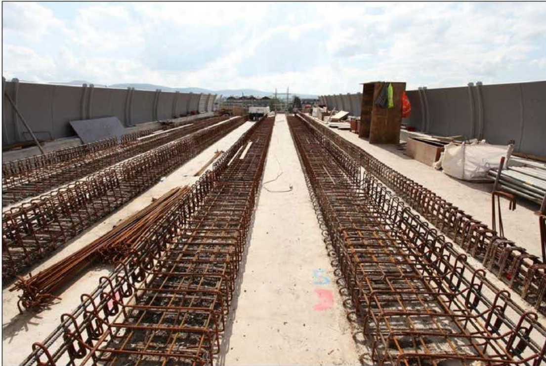
Carricknowe Bridge Trackworks
