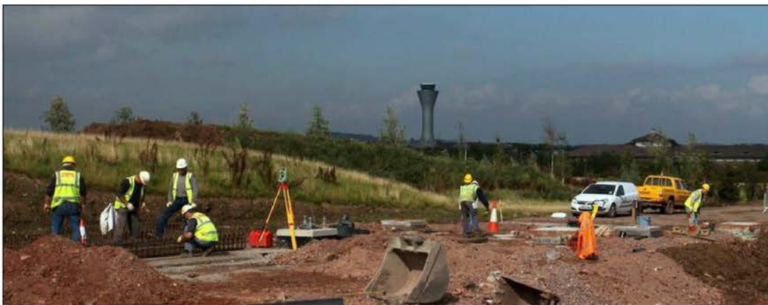
Section 7 Trackworks Setting Out
