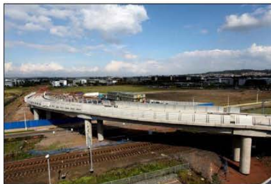
Edinburgh Park Viaduct
