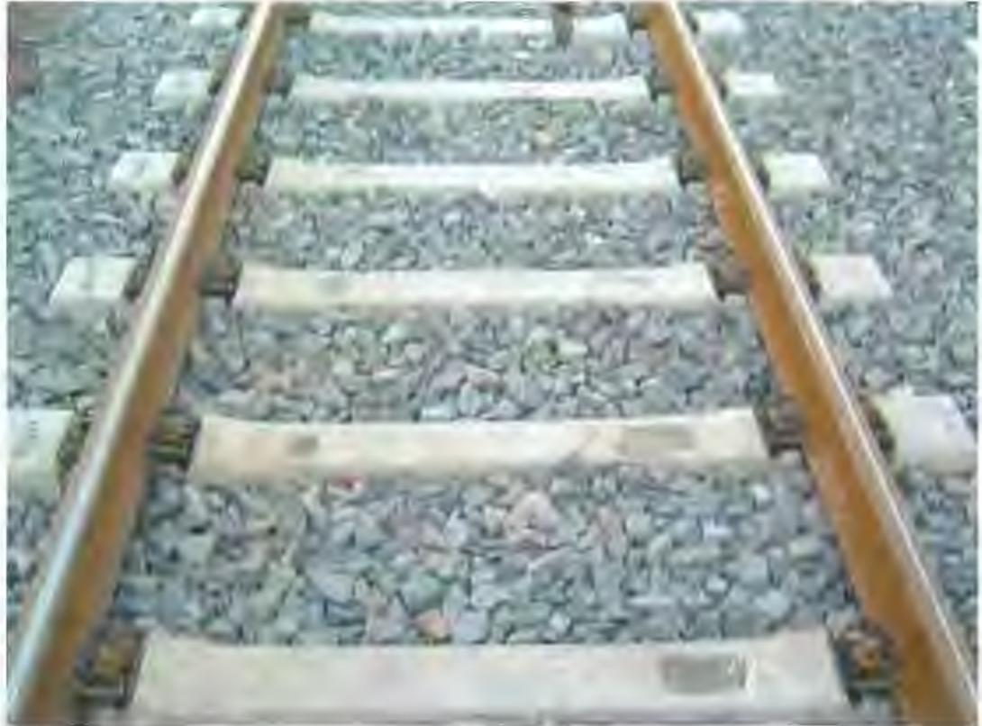
*Figure: Example for Ballasted Track*
