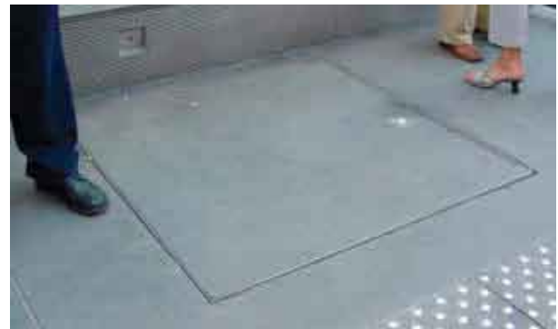
UNDERGROUND EQUIPMENT, LYON
