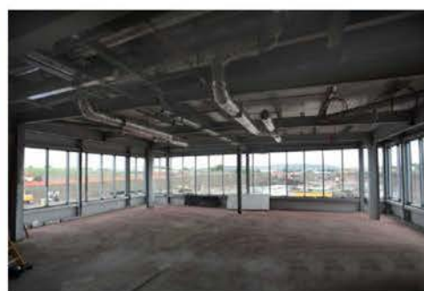
Gogar Depot Control Room
