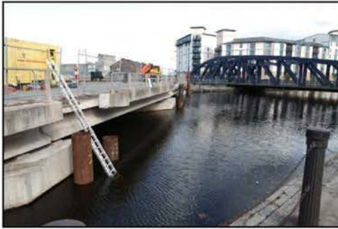
Tower Place Bridge Piling Works
