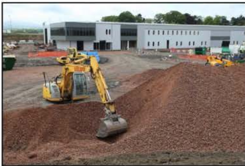
Gogar Depot External Works
