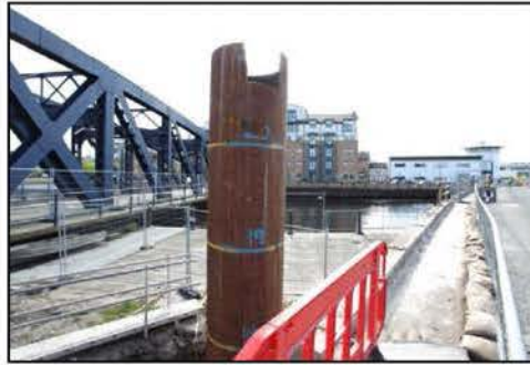
Tower Place Bridge Piling Works
