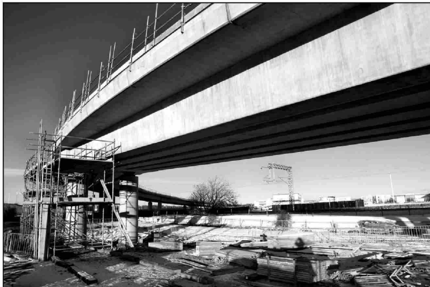
Edinburgh Park Viaduct
