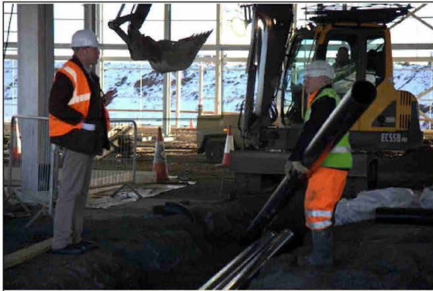
Gogar Depot Internal Works
