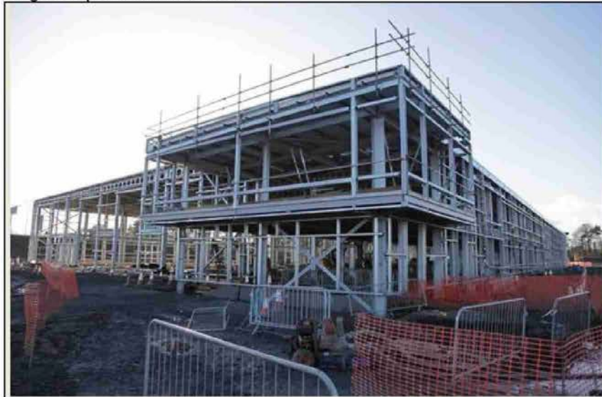
Gogar Depot External Works
