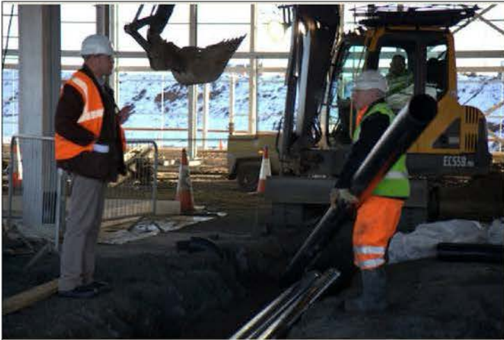
Gogar Depot Internal Works
