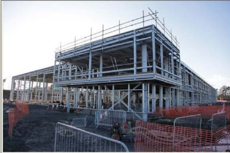
Gogar Depot External Works
