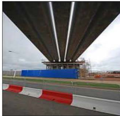
Bridge beams installed at Edinburgh Park viaduct
