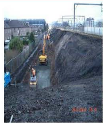
Baird Drive Embankment Construction
