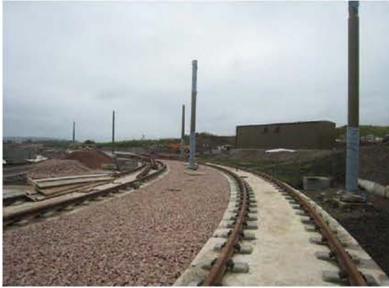
Track work at new Ingliston
