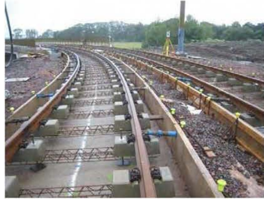
Track work at Gogar landfill Site
