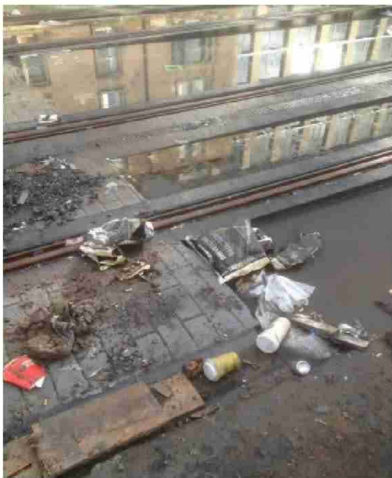
Poor housekeeping – Clifton Terrace
