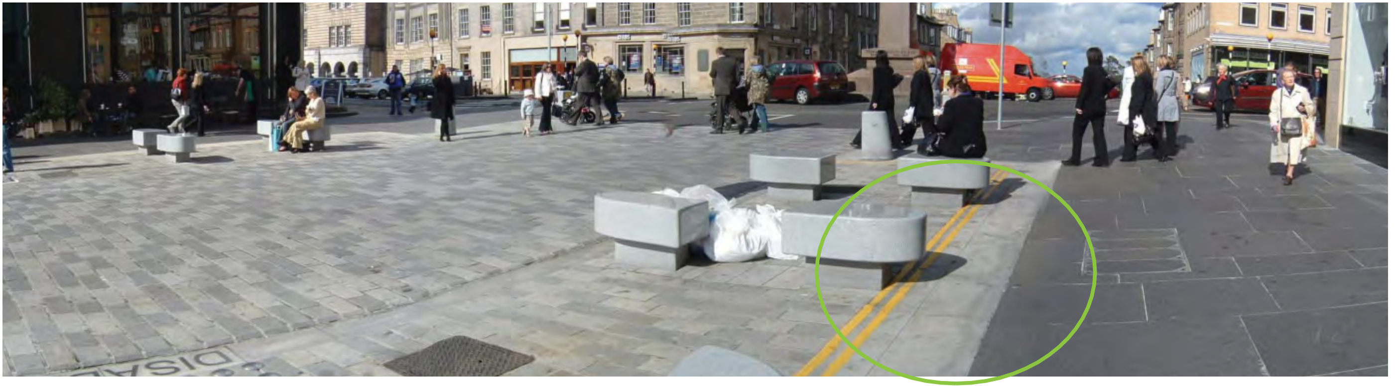
▲ Photo 1 : Historic carriageway and footway relationship maintained despite flush street surface
