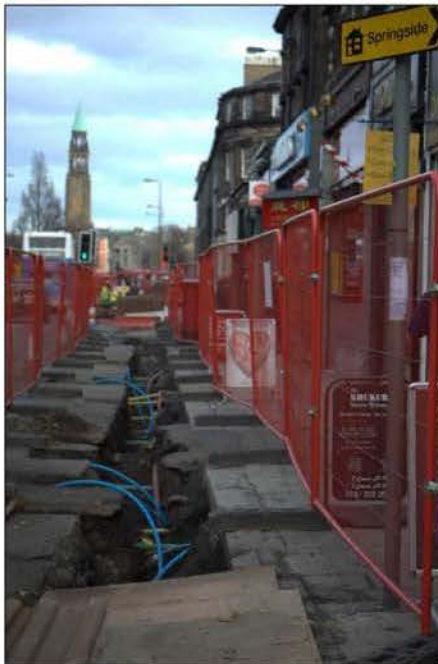
Utilities Diversions – West Maitland Street
