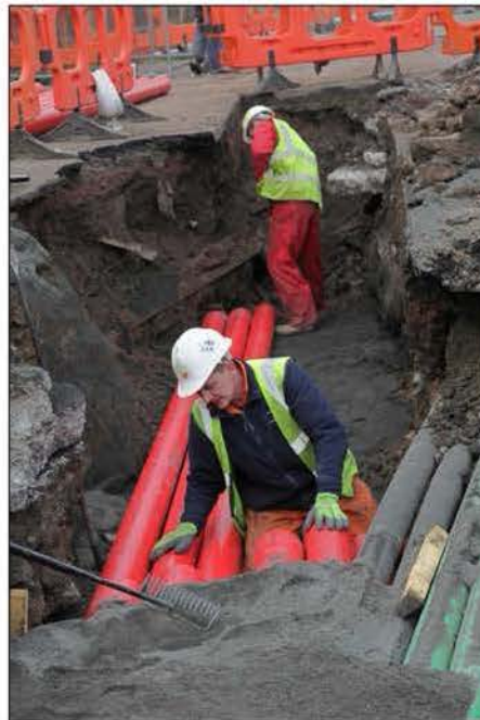
Utilities Diversions at Broughton Street
