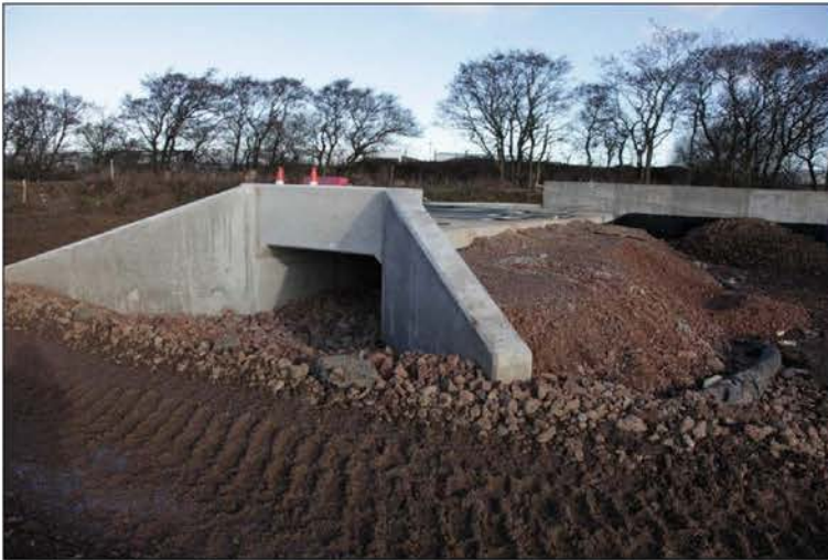
Section 7 Gogar Culvert
