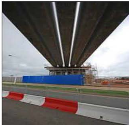
Bridge beams installed at Edinburgh Park viaduct
