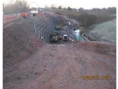
Soil Nailing at Gogar Embankment
