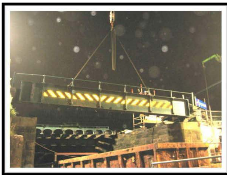
Removal of the existing Network Rail Access Bridge - Balgreen Road
