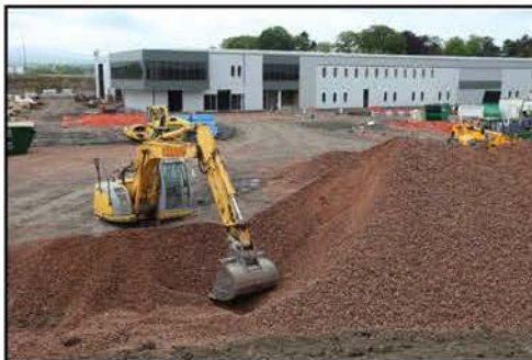
Gogar Depot External Works
