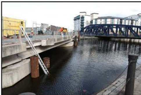
Tower Place Bridge Piling Works
