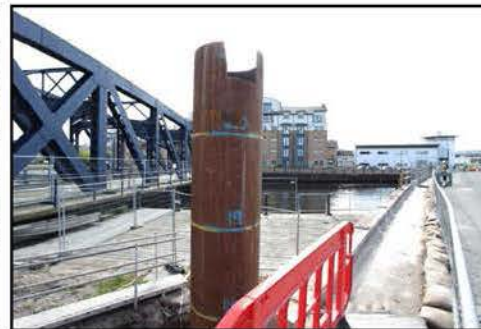
Tower Place Bridge Piling Works
