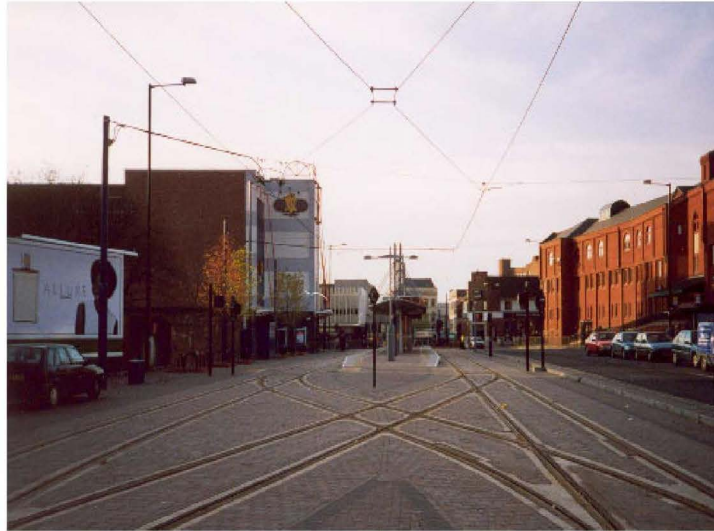
Figure C.12: Typical Overhead Line Equipment (OLE) Wolverhampton Midland Metro
