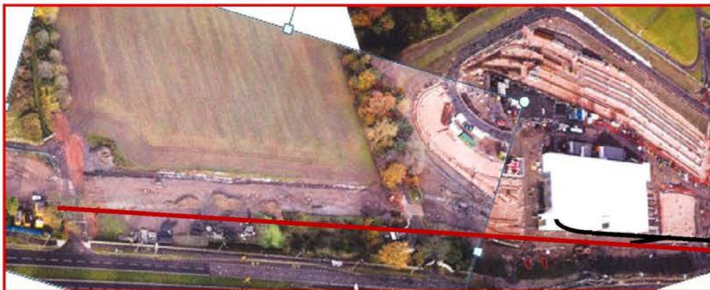
Figure 2. Aerial Photo - the Mini-test track
