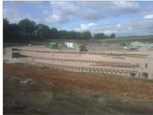
Track Progress at Gogar Dept
