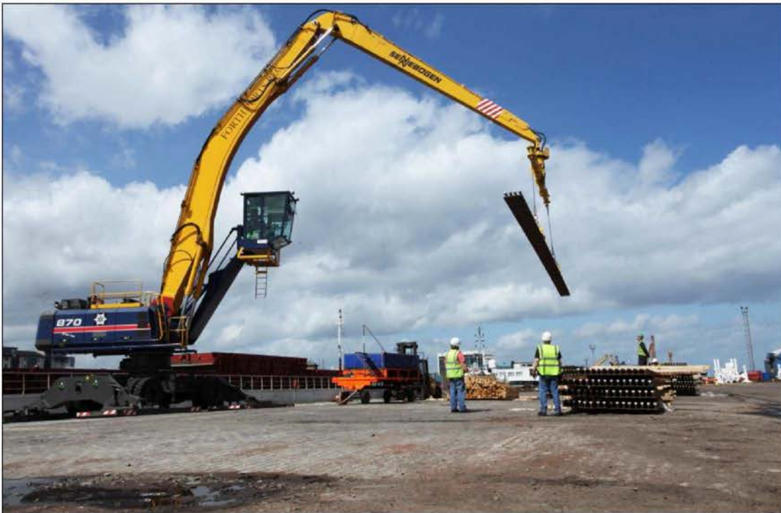
Rail Delivery Leith Docks
