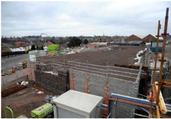
- Murrayfield Tram Stop Light weight Aggregate Fill
