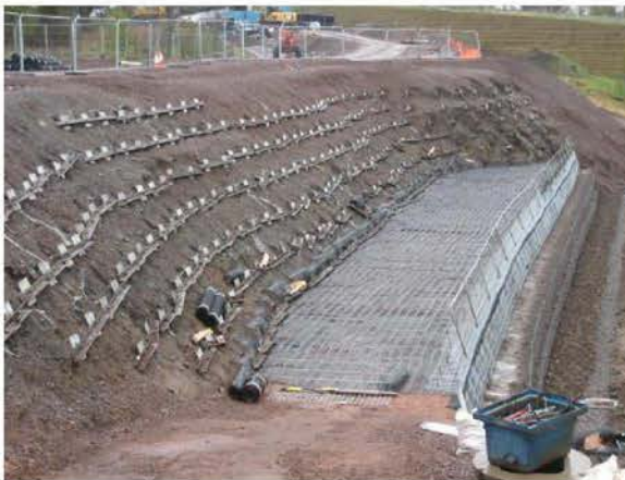
- Soil Reinforcement – Gogar Landfill Site
