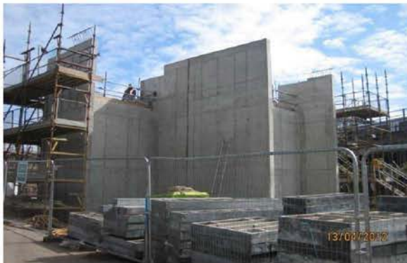
- West Abutment S504
