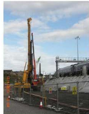
W3 Piling Operations
