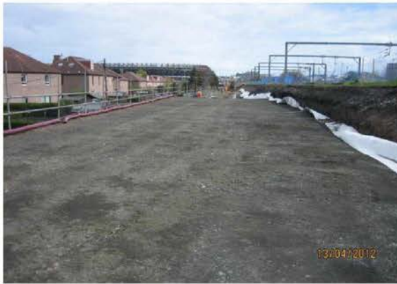
- Baird Drive – reinforced earth embankment
