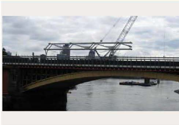
1st section of roof spine beam installed
