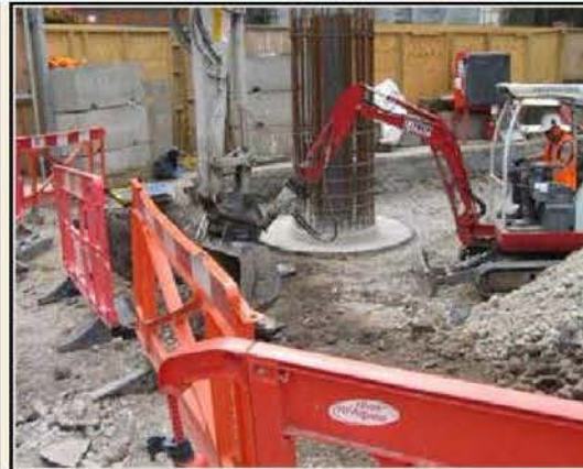
Rebar Installation to Column K in 3 Crown Sq
