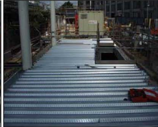
Turnmill Concourse formwork
