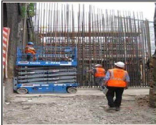
Steel Fixing to Wall B at Park St.
