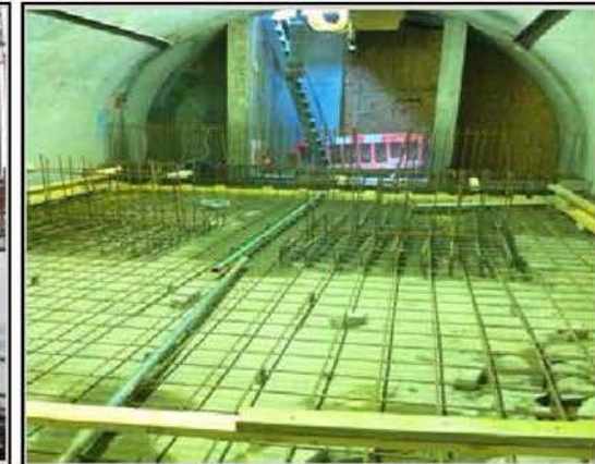
Slab & Anchor Block Steelwork in RA Vault 8
