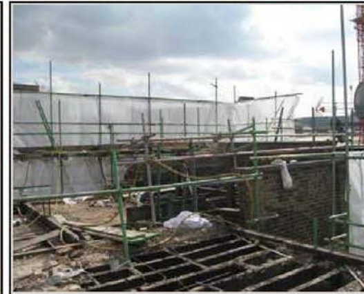
Ongoing Demolition of 3rd Floor to 11-15 BHS
