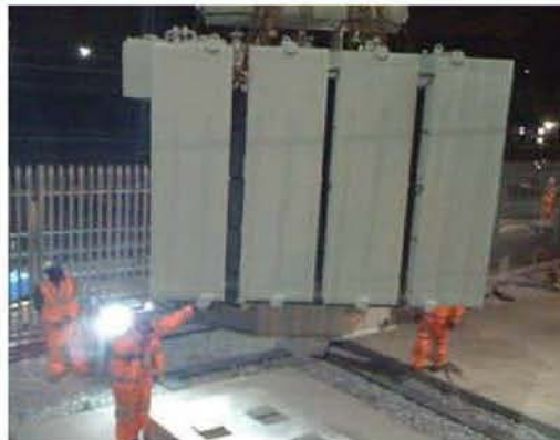
Auto Transformer lifted into position on plinth
