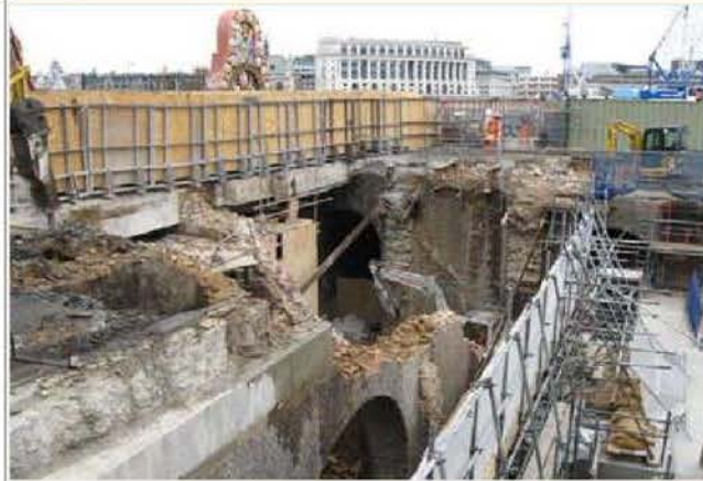
South Station demolition progressing
