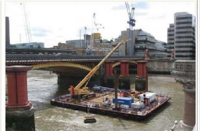
100T Barge Crane in position
