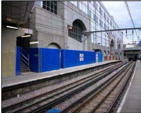
Platform 4 - New Hoarding installation
