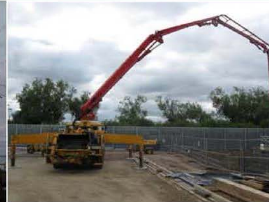
E&P Concrete pumping into Disconnecter base
