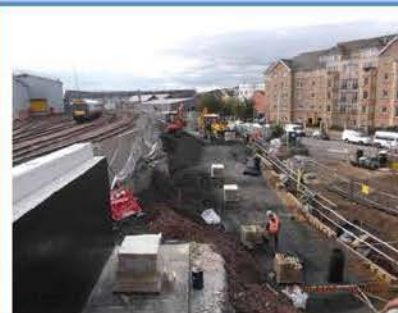
W3 Retaining Wall, Russell Road
