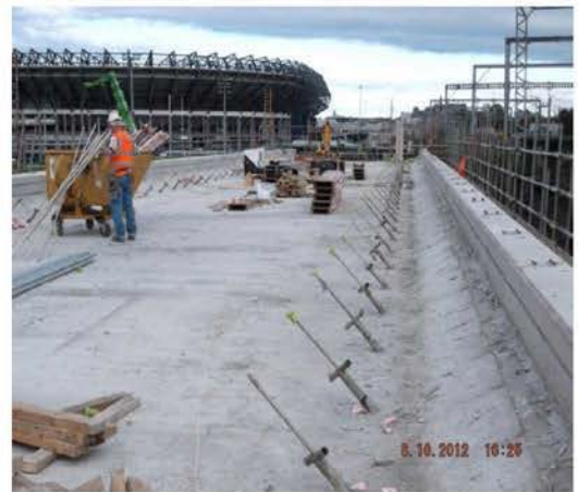
Water of Leith Bridge Deck
