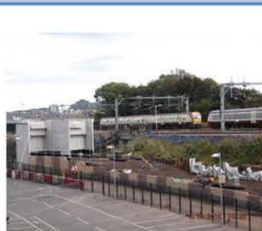
S505 Earth Retaining Wall, Murrayfield
