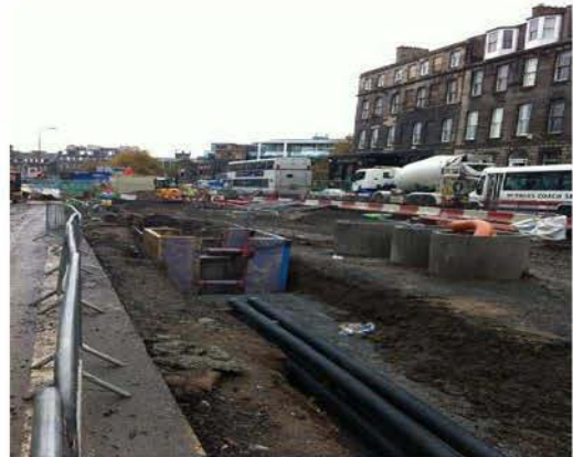
Drainage York Place
