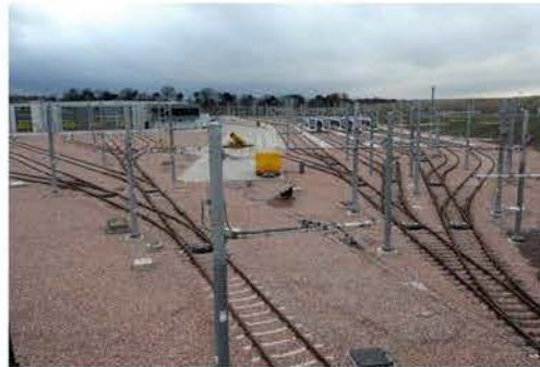
View of the Depot from the access bridge
