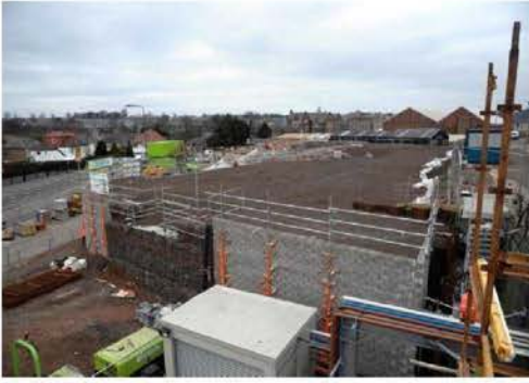
- Murrayfield Tram Stop Light weight Aggregate Fill
