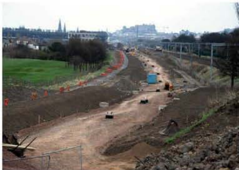
- Carricknowe to Balgreen Bridge
