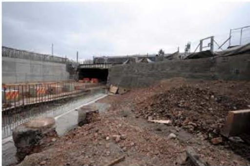
- Russell Road Bridge
