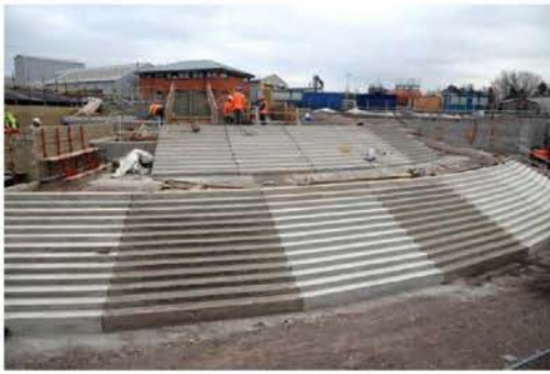
- Murrayfield Tram Stop Steps
