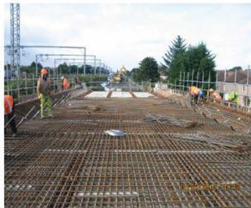
The deck construction at the Water of Leith.
