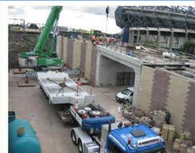
Roseburn Precast Track Slab Units
