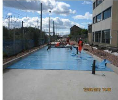
Floating trackslab being installed at Haymarket Yards
