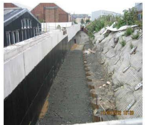
W3 and W4 wall construction continuing;
