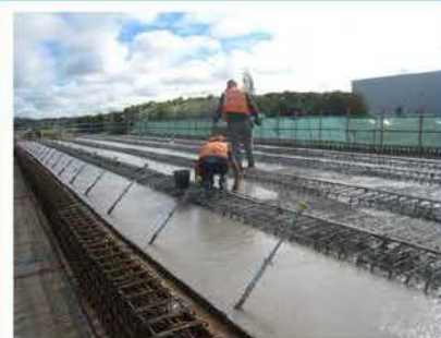
South Gyle Access Bridge Deck Poured
