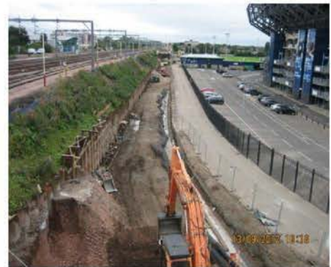
Tensar wall construction at S21B Murrayfield commencing
