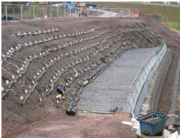
- Soil Reinforcement – Gogar Landfill Site
