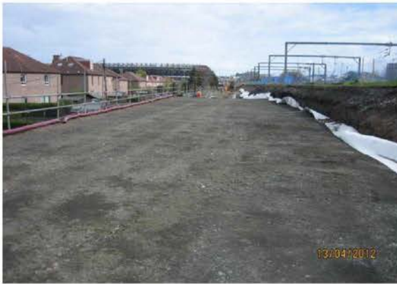
- Baird Drive – reinforced earth embankment
