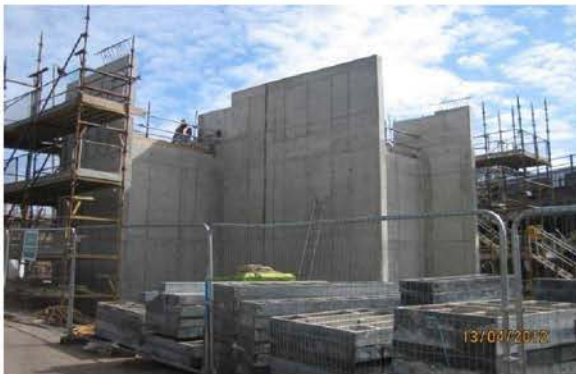
- West Abutment S504
