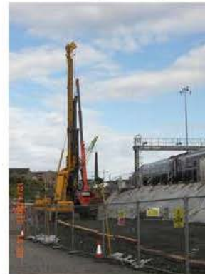
W3 Piling Operations
