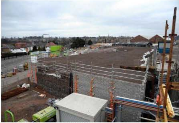
- Murrayfield Tram Stop Light weight Aggregate Fill
