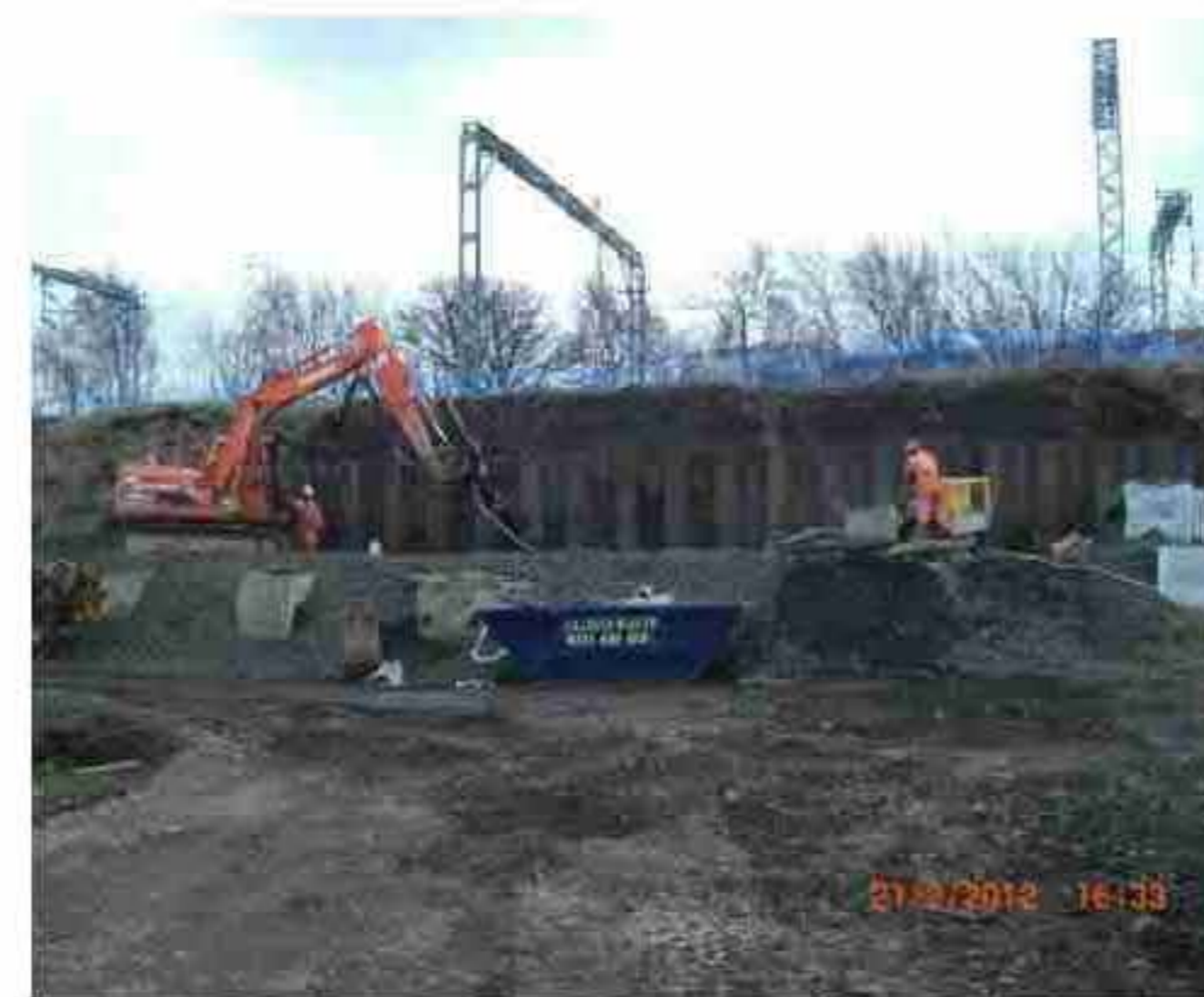
Water of Leith Abutment Construction
