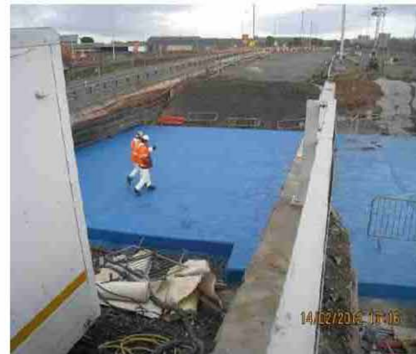
A8 Underpass Waterproofing
