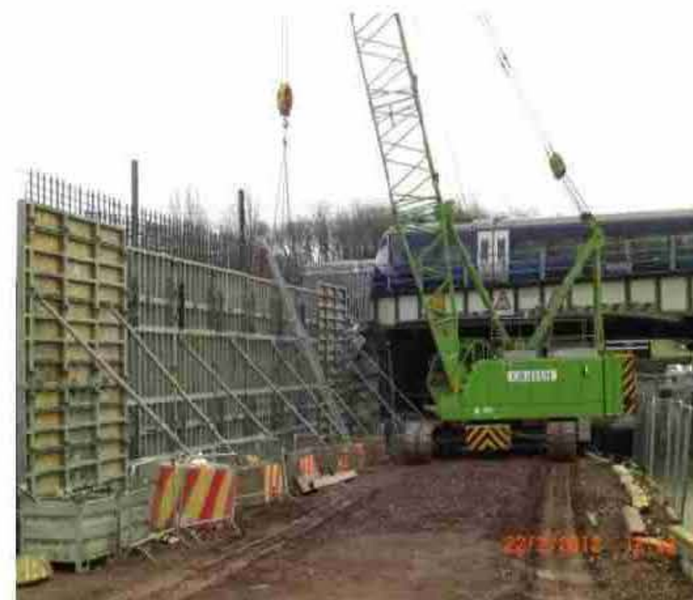
Russell Road Bridge Abutment Construction
