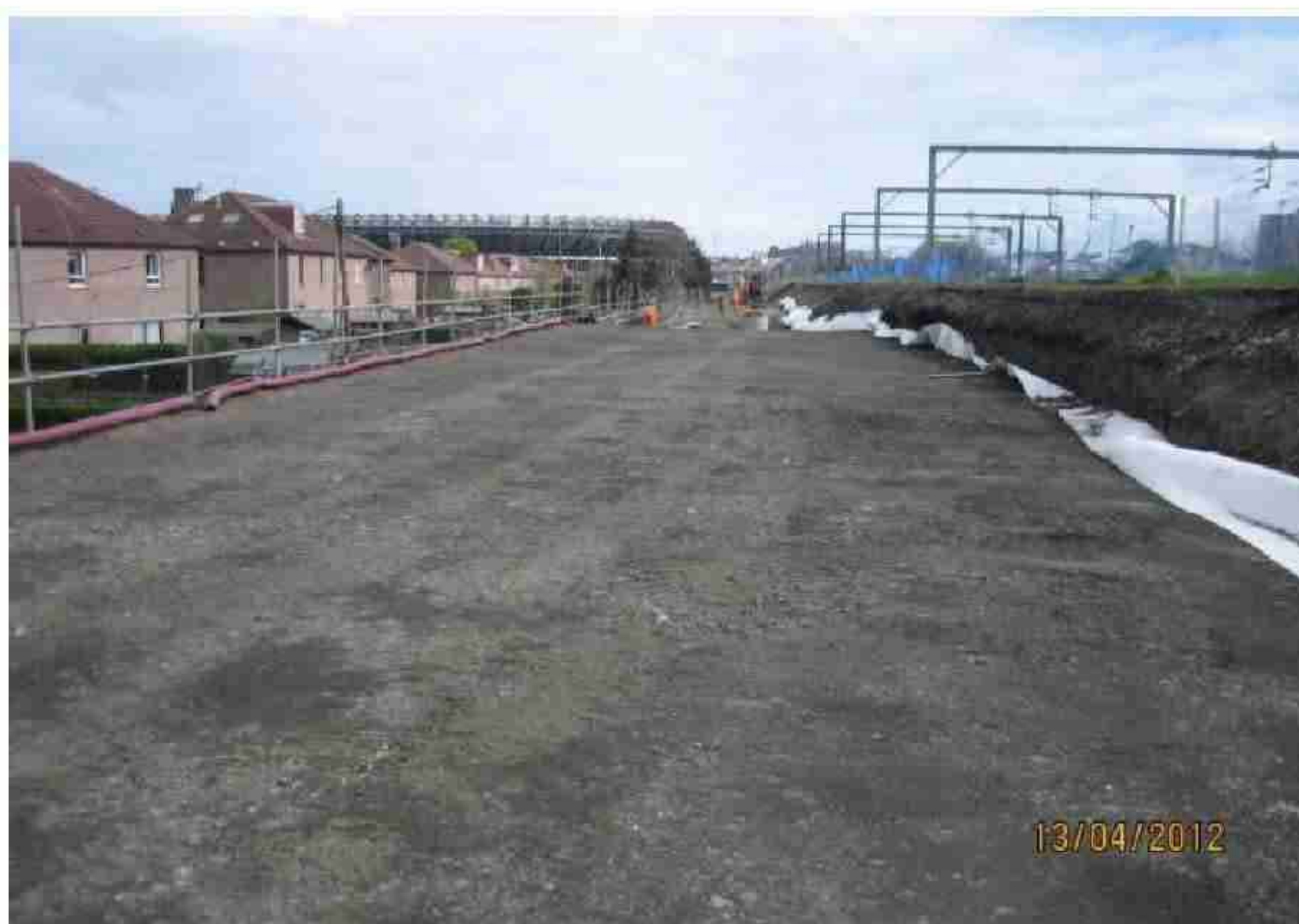
- Baird Drive – reinforced earth embankment
