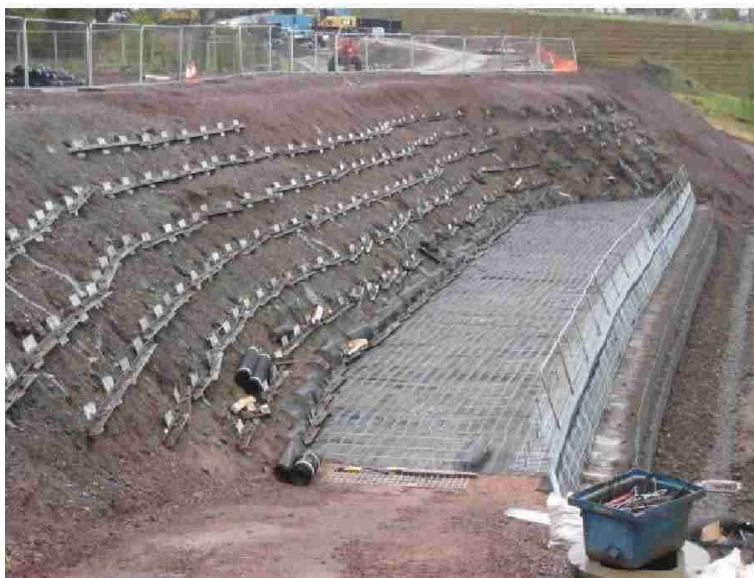
- Soil Reinforcement – Gogar Landfill Site
