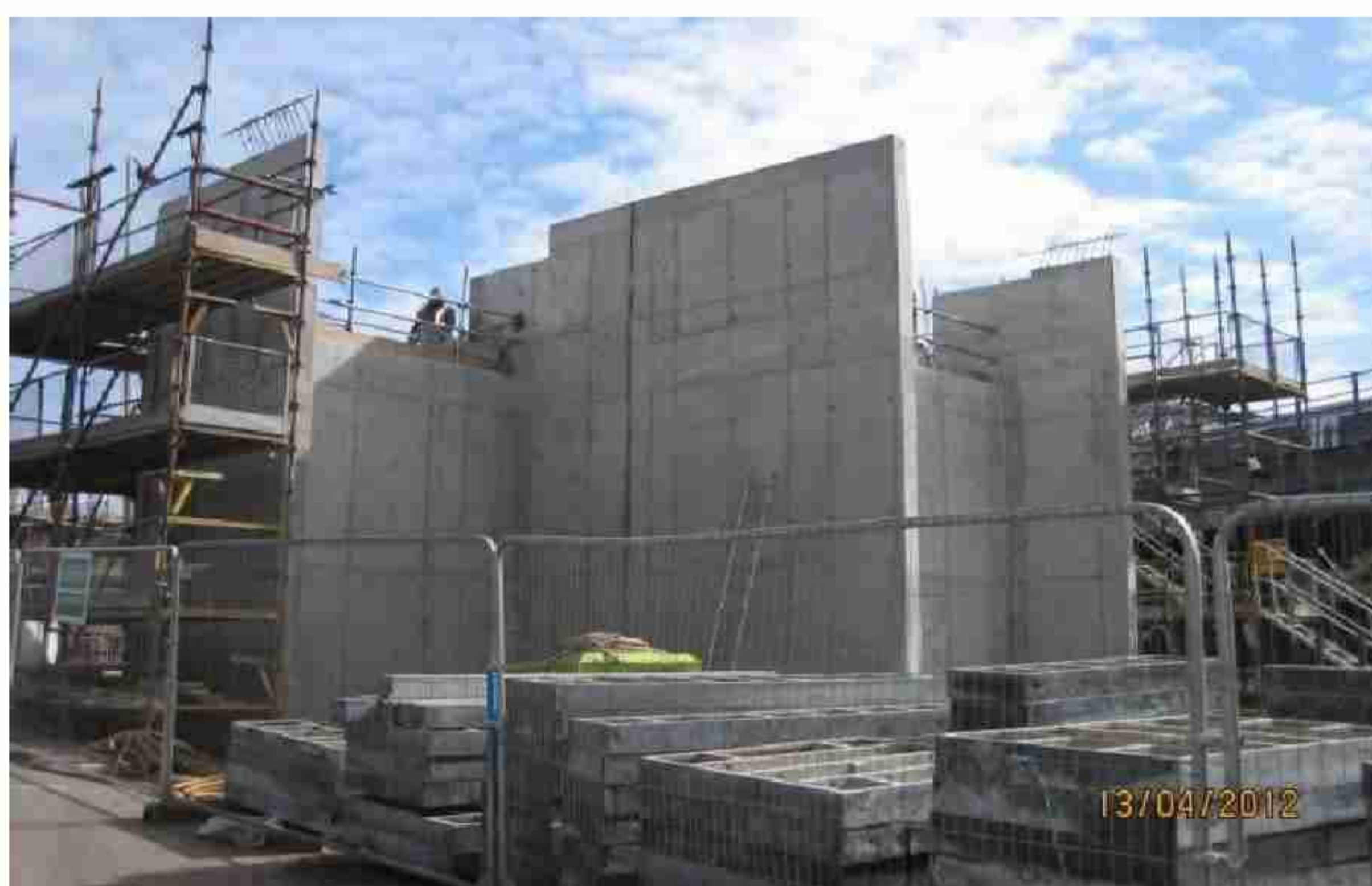
- West Abutment S504
