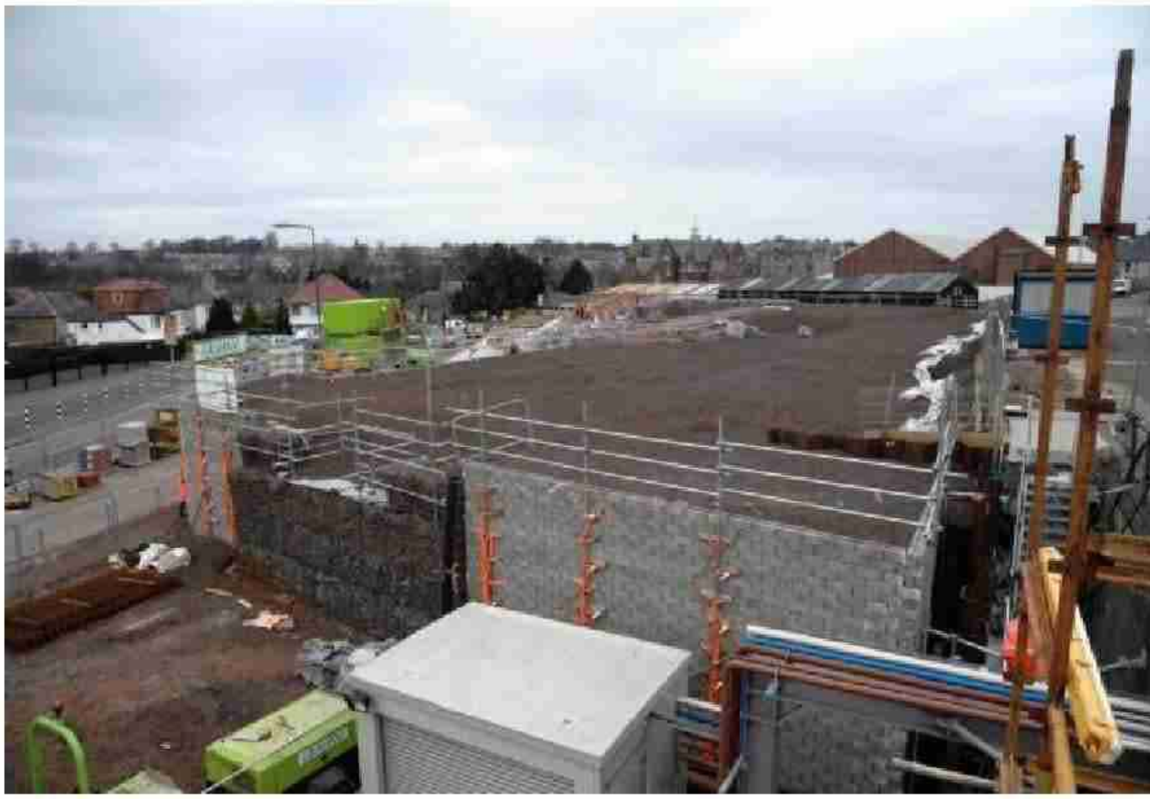
- Murrayfield Tram Stop Light weight Aggregate Fill
