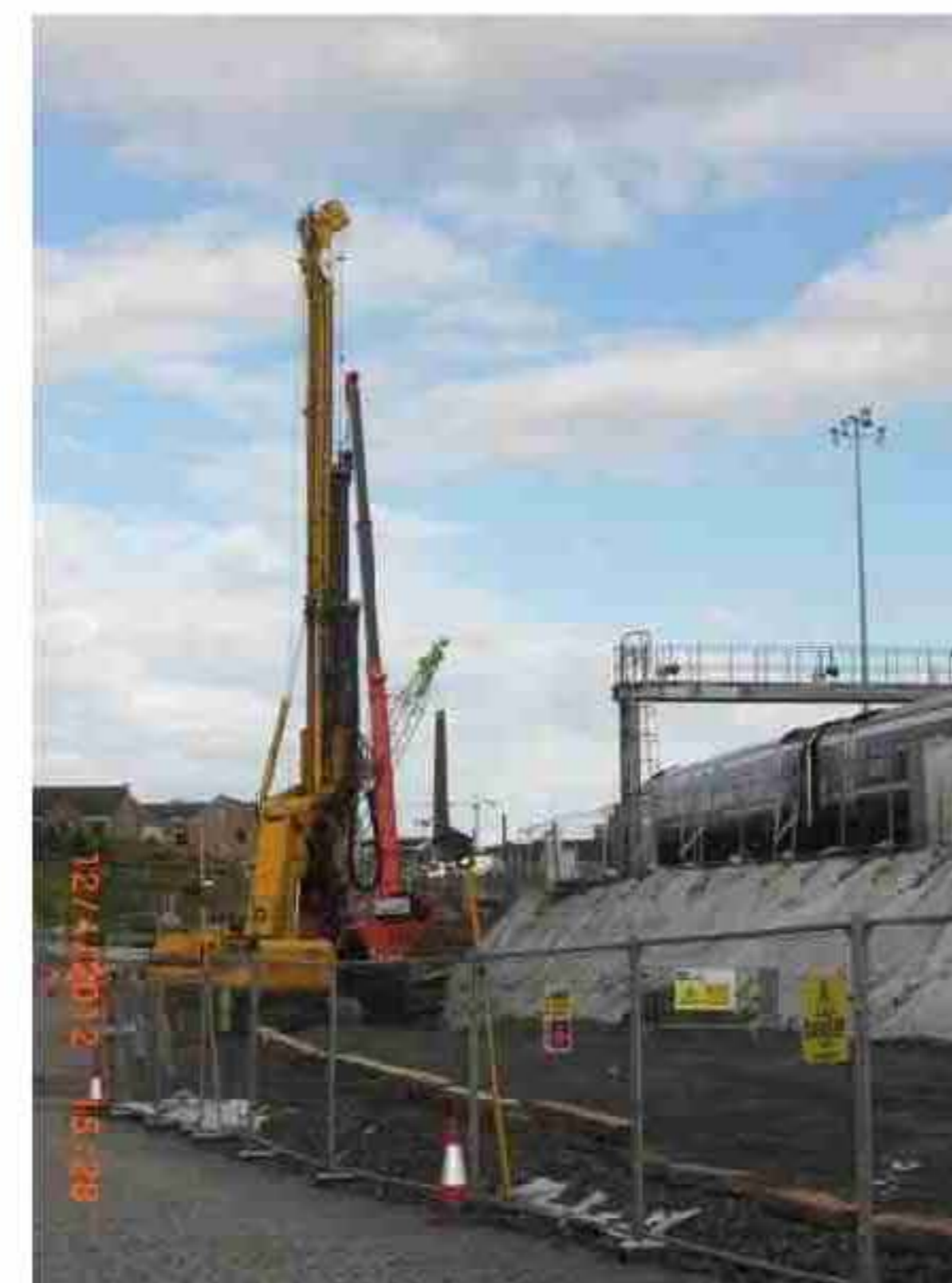
W3 Piling Operations
