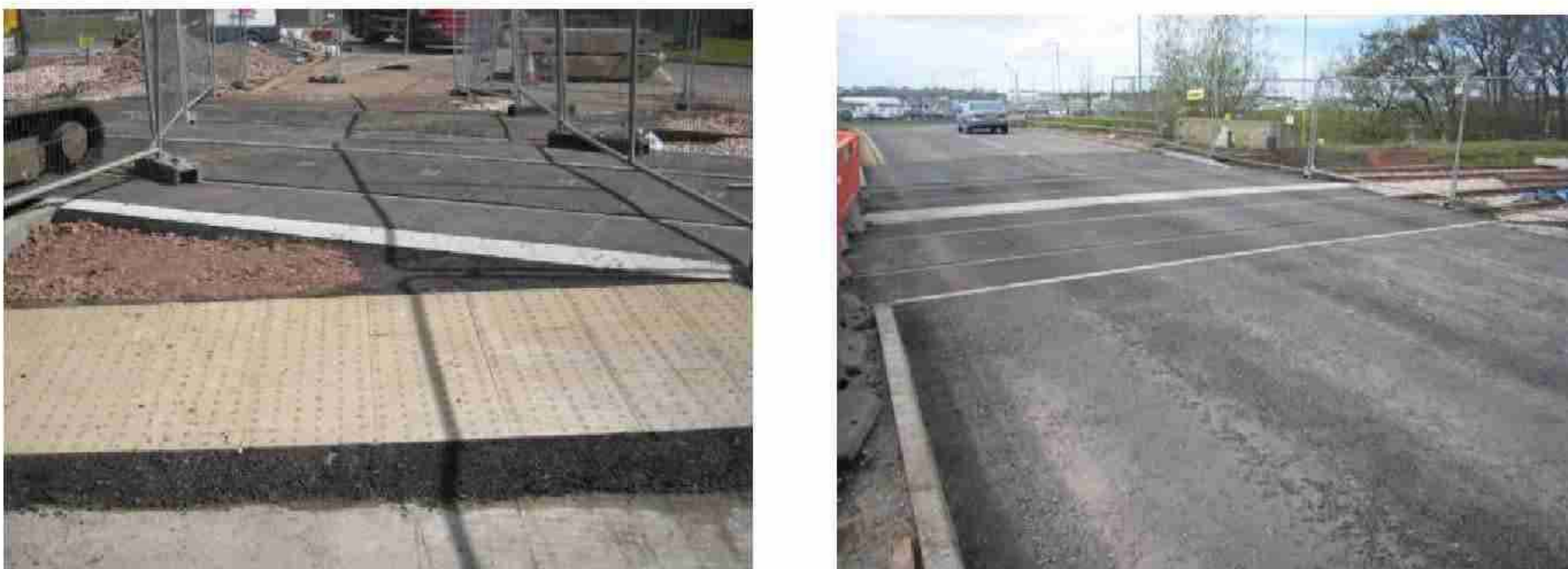
Photos: Eastfield Avenue Pedestrian and Road Crossing
