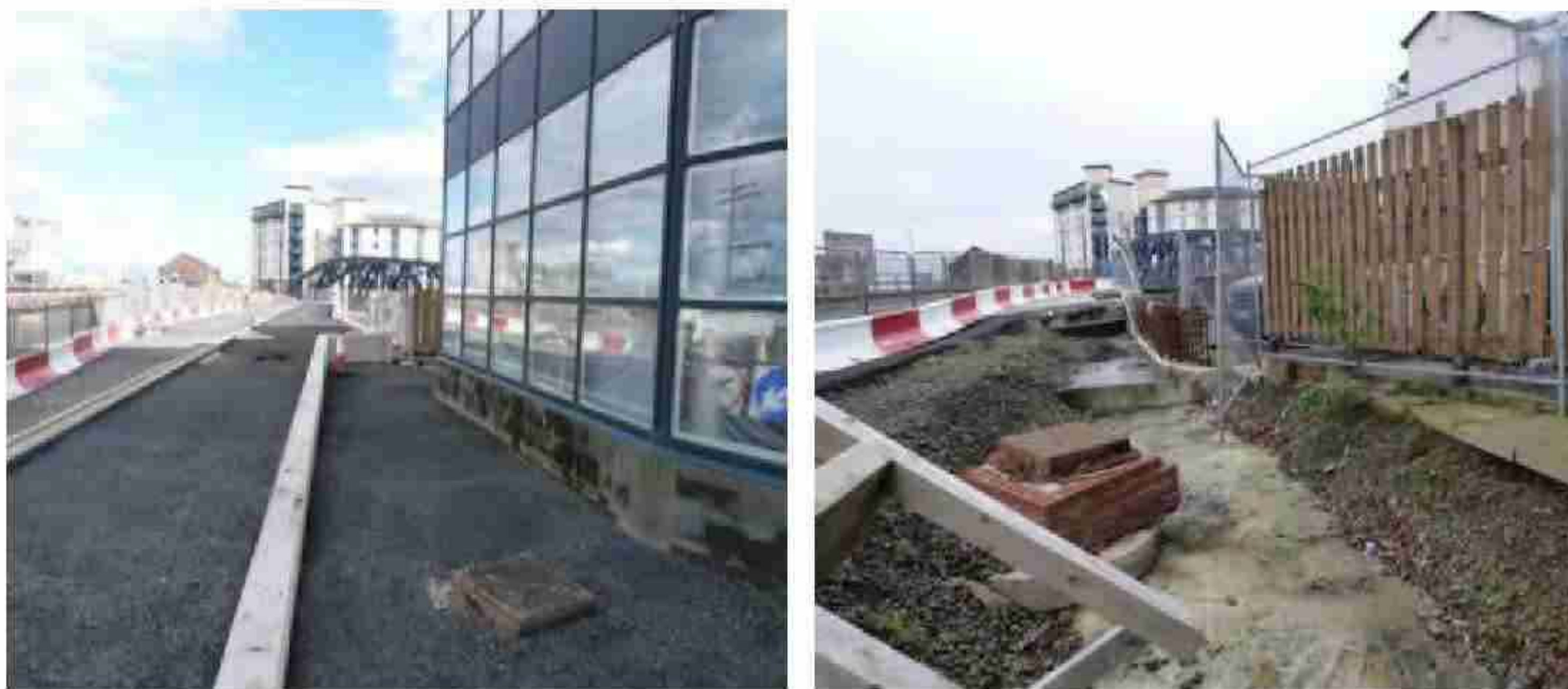
Tower Place Bridge nearing completion
