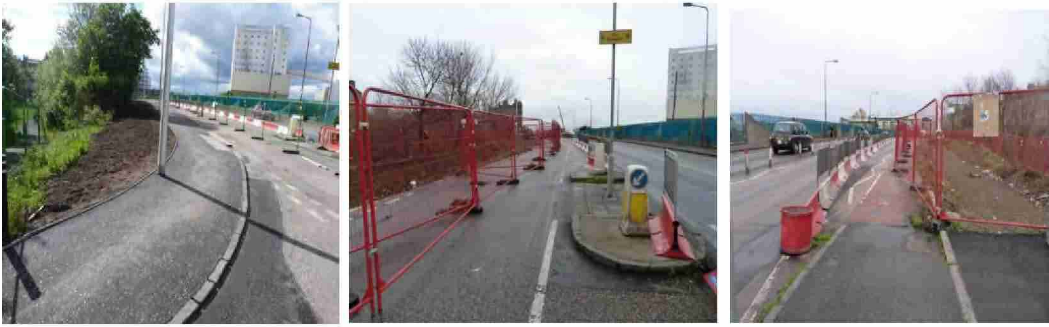
Lindsay Road nearing completion
