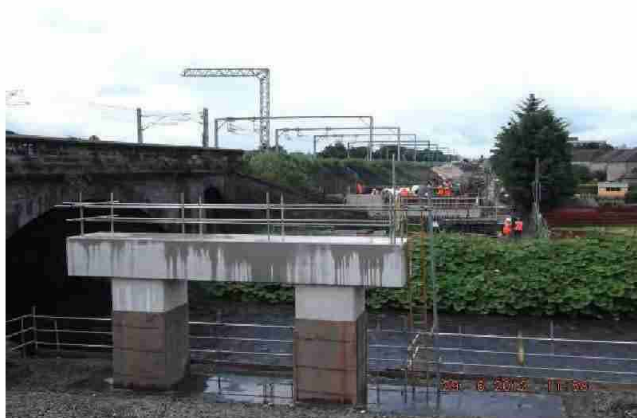
Water of Leith Bridge Abutment
