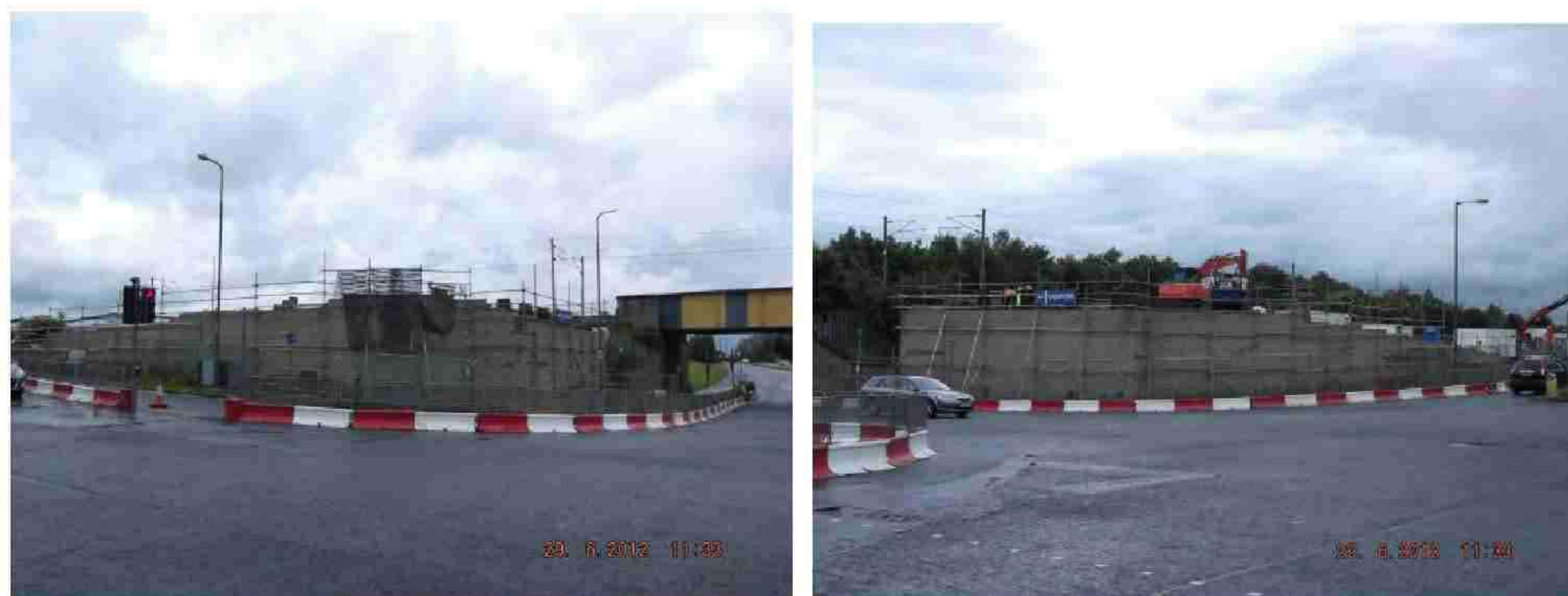
South Gyle Access Bridge Abutment Construction
