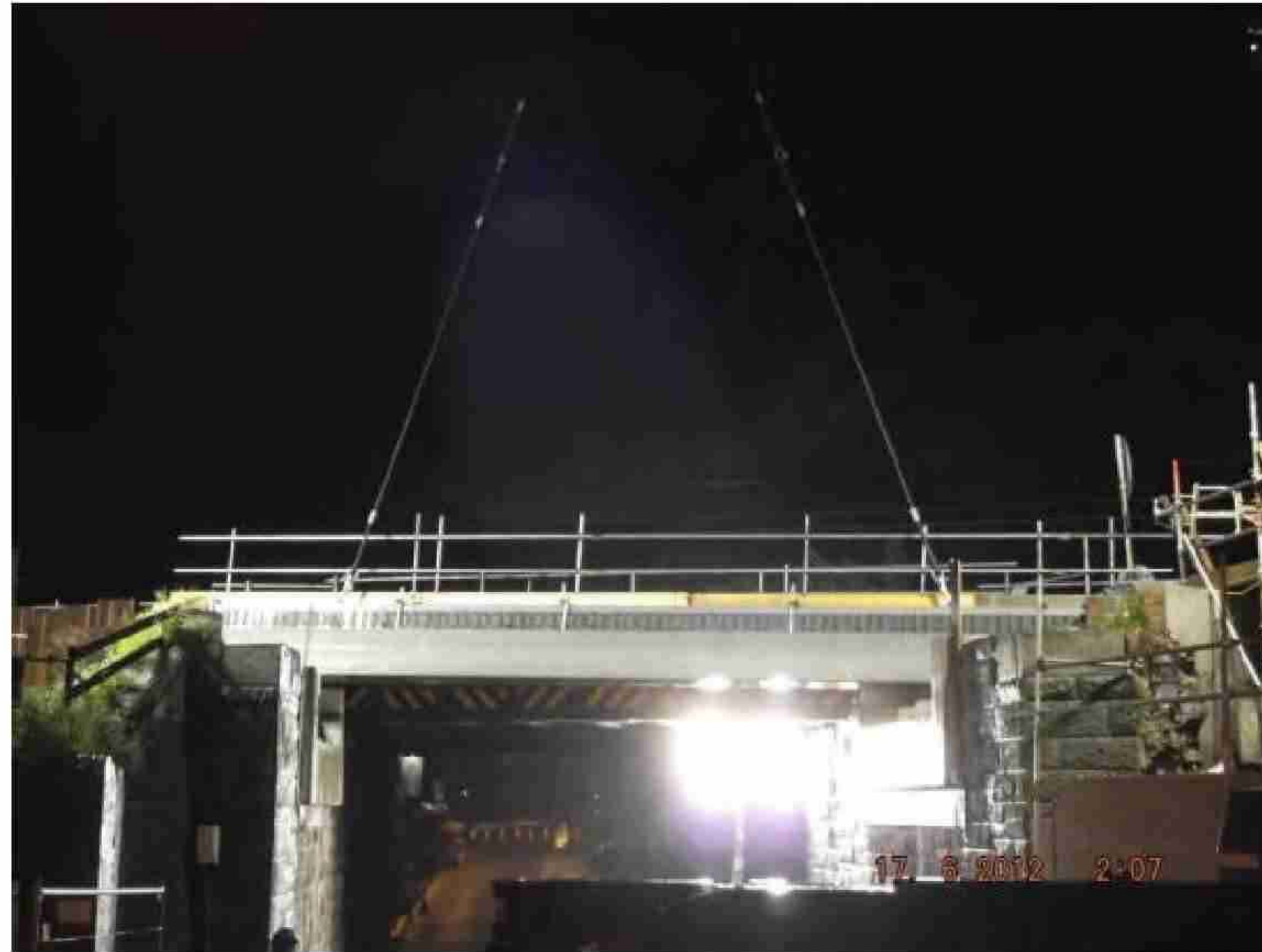
Balgreen Bridge Beam Installation
