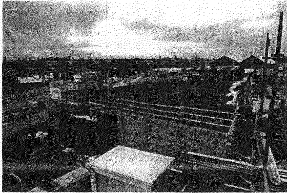
- Murrayfield Tram Stop Light weight Aggregate Fill
