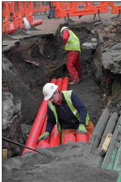
Utilities Diversions at Broughton Street
