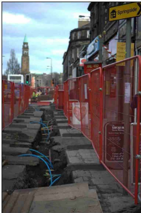
Utilities Diversions – West Maitland Street
