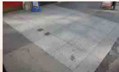
Block of grey concrete paving laid across the footway
