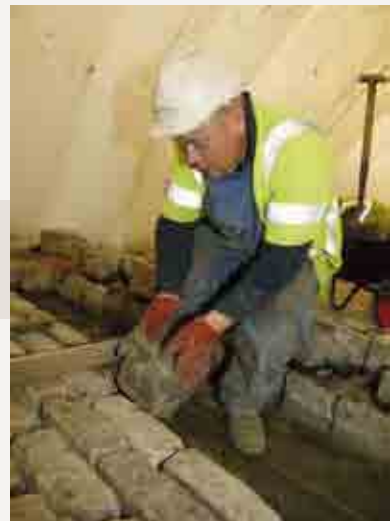
Laying reclaimed stone setts
