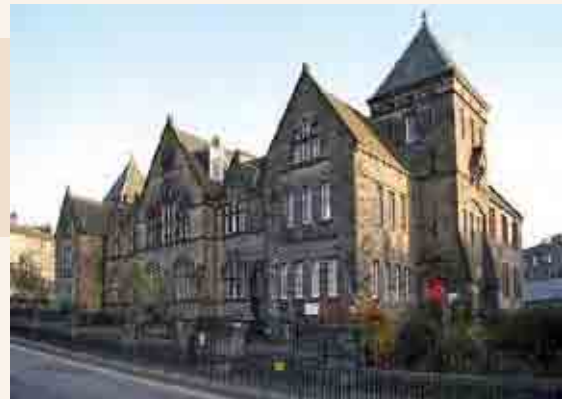
Guard rail / visi rail used as safety precaution outside primary school
