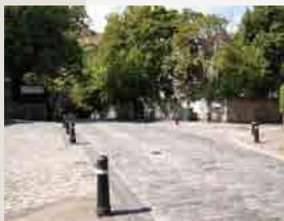
Reclaimed sett surfacing
