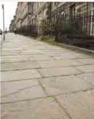
Paving laid 90° to kerb
